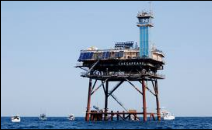
Figure 9: Chesapeake Light Offshore Monitoring Station (43m Above MSL Meteorological Tower)
