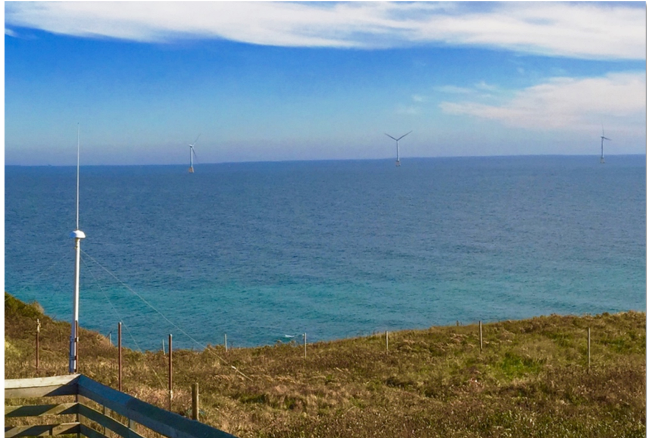
Block Island 5-turbine array, installed 2016
