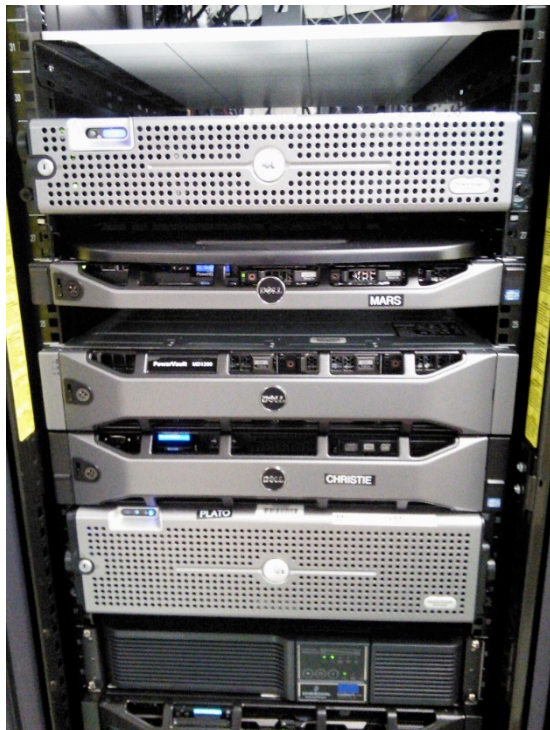
Figure 10: Photo of the disk storage hardware installed on the campus of Stevens Institute of Technology.
