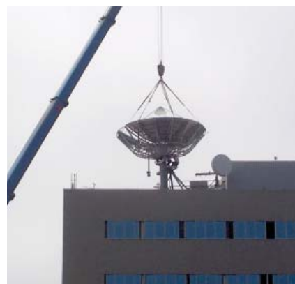
HiSeasNet antenna installation on the SDSC roof
